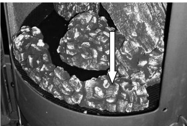
6. Slide the Right front ember strip next to the Left ember strip. The two fit together to hide the seam.
